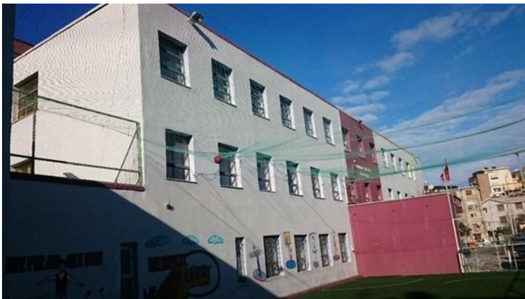
Figure 9. The main building under investigation.
