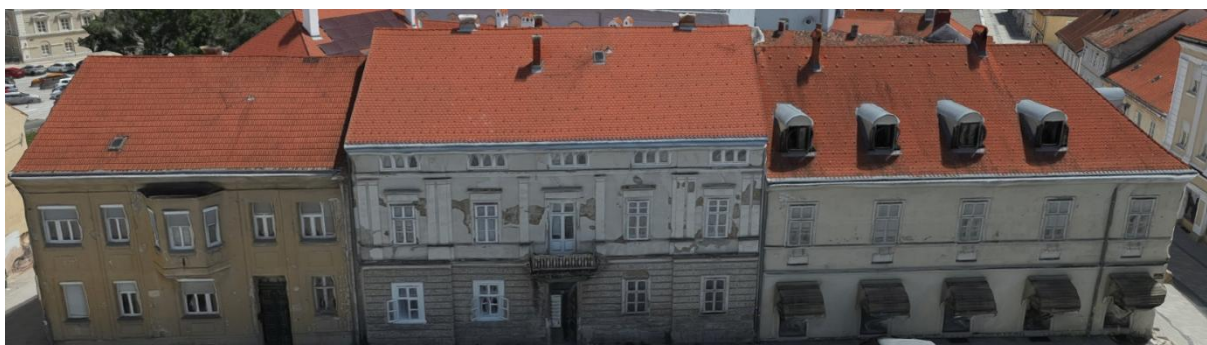
Figure 7. A detailed photogrammetric model of three representative buildings within the surveyed zone.
